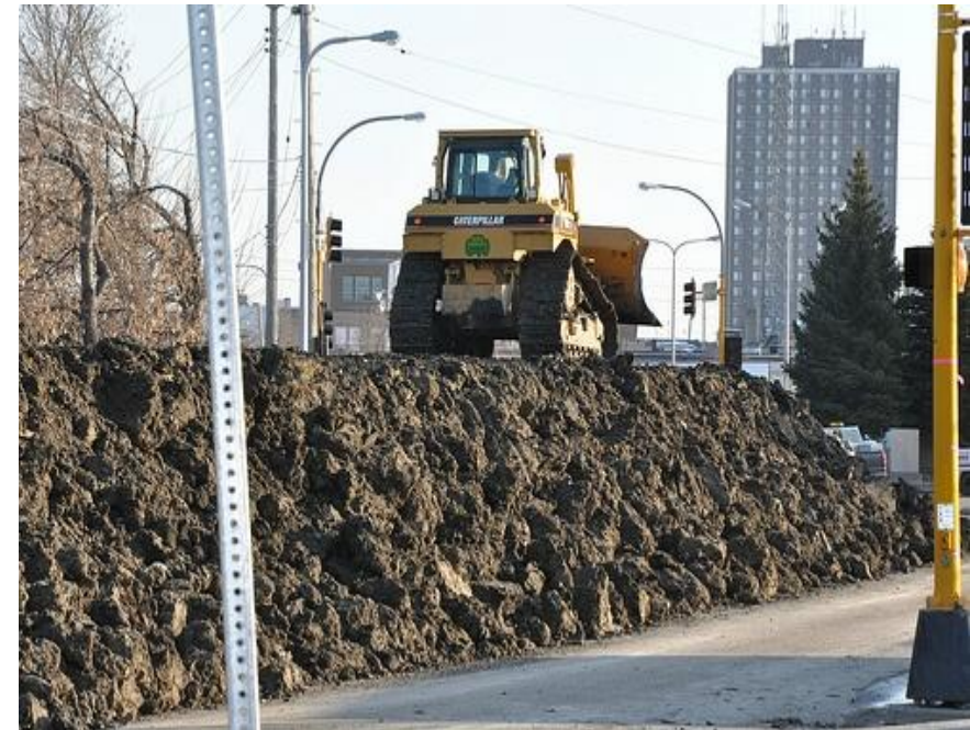
Building of 2 nd St. Levee for 2009 Fargo-Moorhead Flood
