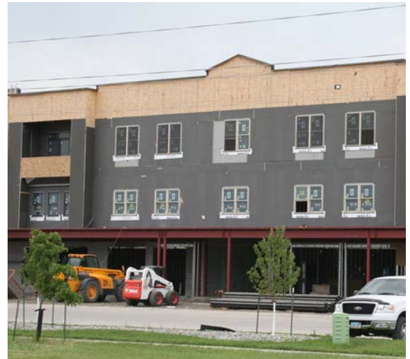
A Mixed-Use project under construction in Fargo.
