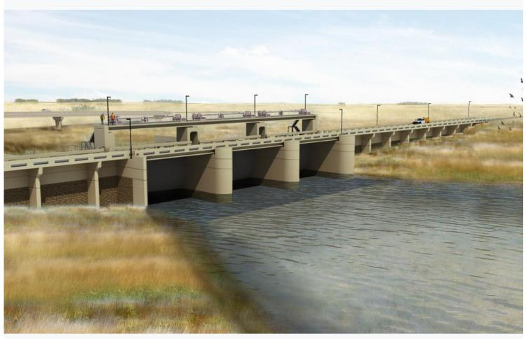
This is a rendering of the Fargo-Moorhead flood diversion's dam inlet structure planned for near Horace, N.D., looking downstream. The inlet controls the flow of water from the dam into the diversion channel to reduce impact
