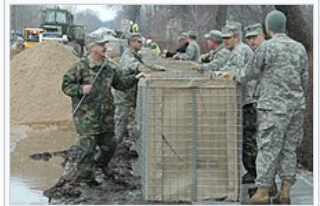
HESCO collapsible barriers were used to prevent flooding
