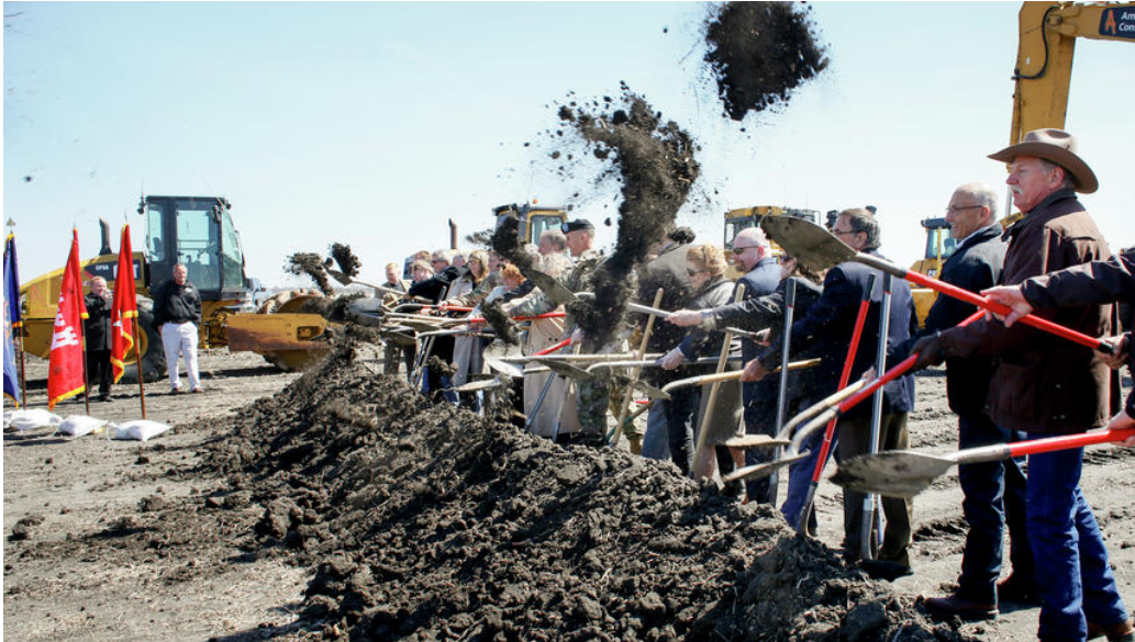
The Fargo-Moorhead Diversion Authority and U.S. Army Corps of Engineers officials break ground Monday, April 17, 2017, on the flood diversion at the site of the dam inlet structure south of Horace, N.D. Michael Vosburg / Forum Photo Editor
