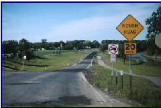
Pavement patches to remediate recent rifting are apparent in this photo taken in August, 1997. View is toward the north.
