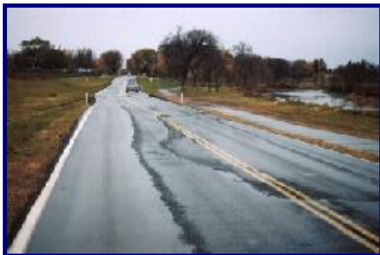
Rifted and uneven pavement of Elm Street. View is facing north toward intersection with 15th Ave. N. (1996). The dike is visible to the left of the photo.
