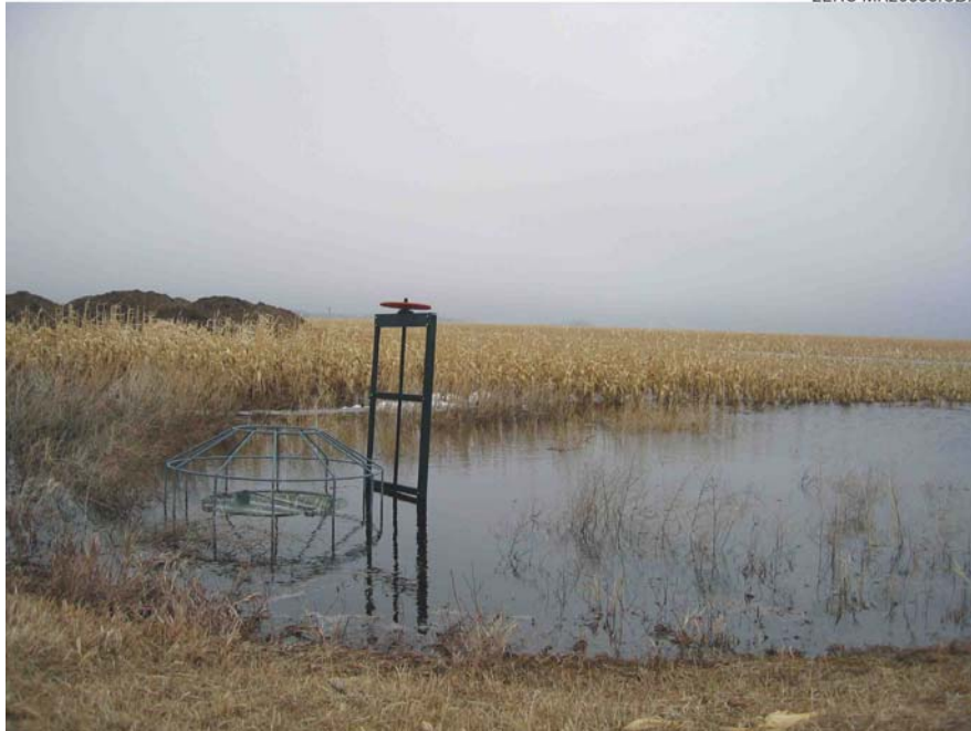
Figure 41. Shelly field trial site at full storage (spring 2005).
