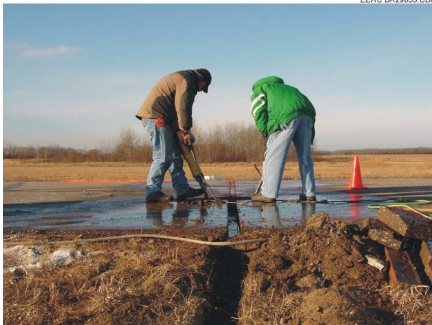
Figure 54. Installation of sensors in cross section of road.
