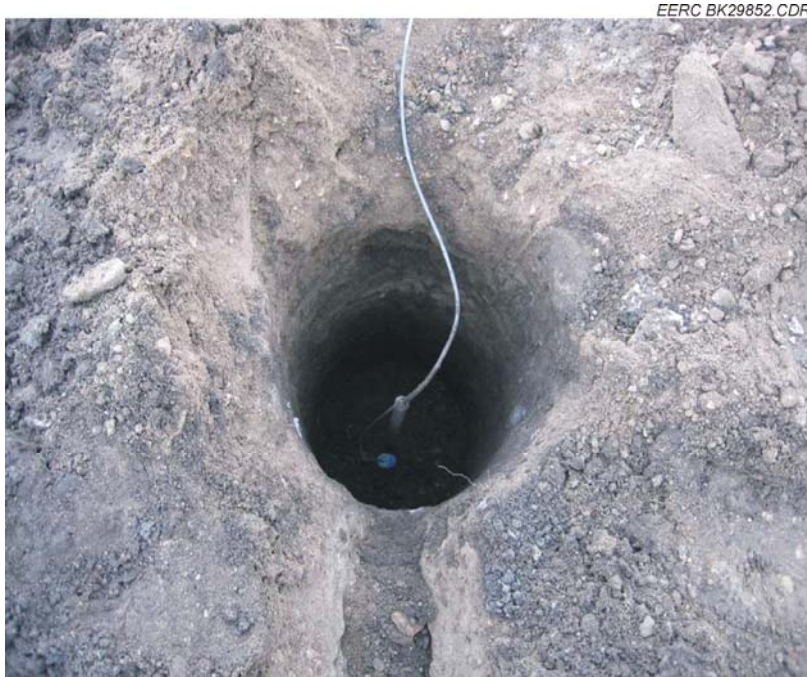
Figure 53. Acrylic rod containing sensors in a borehole within the road.
