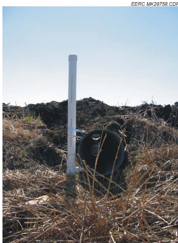
Figure 51. Photograph of stilling well used to monitor culvert water levels.
