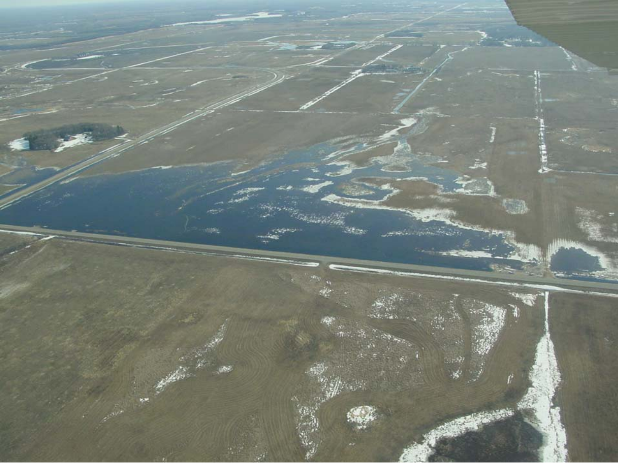
Figure 45. Lake Bronson field trial site at full storage (spring 2006).
