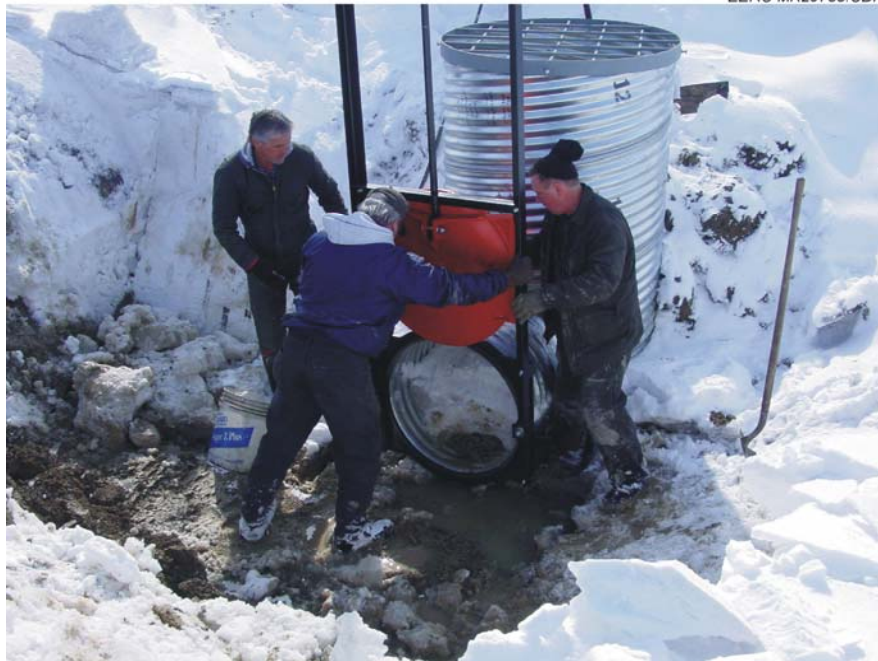
Figure 49. Culvert modification devices (standpipe and canal gate).
