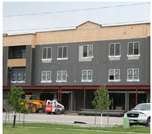
A Mixed-Use project under construction in Fargo.
