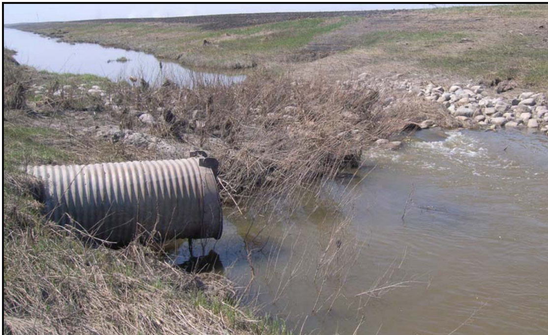
Picture 8 - Rock and culvert structure on the Rush River within the project area. Photo from April 22, 2010.
