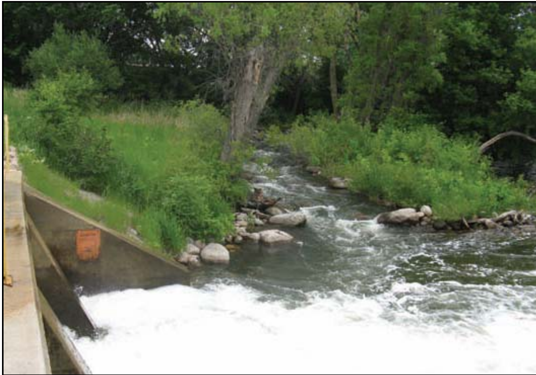
Picture 9 - Example of a fish bypass channel at a dam on the Otter Tail River near Fergus Falls, MN. Project completed in 2002. Photo and information source: Aadland 2002.
