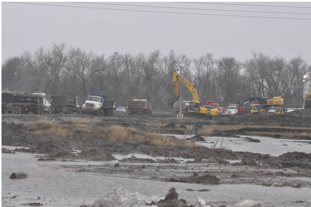
Picture 5 – Agricultural lands, sport facilities, and public areas were dug up for levee material in 2009.
