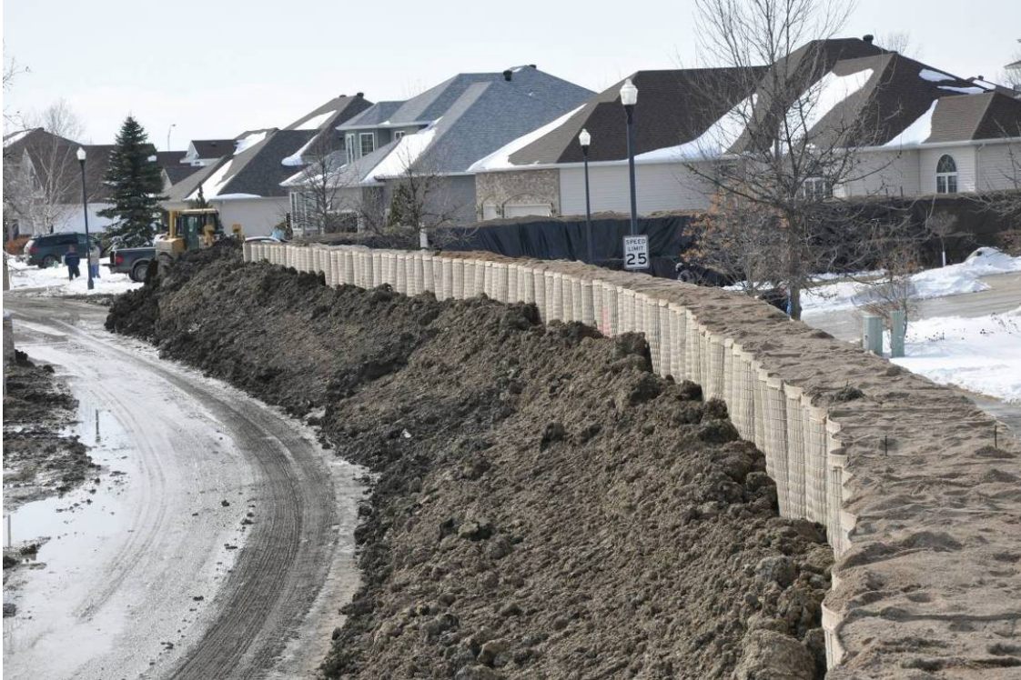
Picture 6 – Sand filled barriers were backed with clay and used as a second line of defense after the sandbags in 2009.
