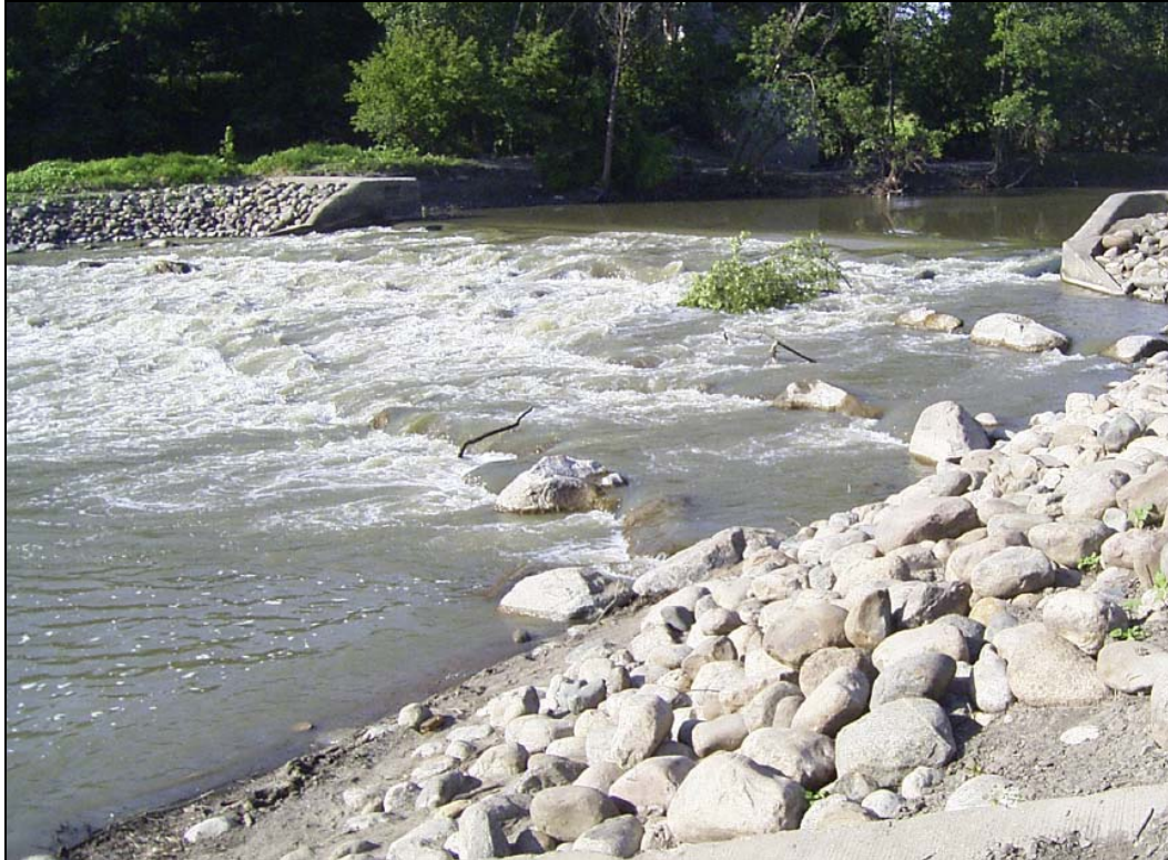
Picture 7 - Example of a rock-rapids fish passage structure at North Dam, Red River of the North, Fargo, ND. Project completed in 2002.
