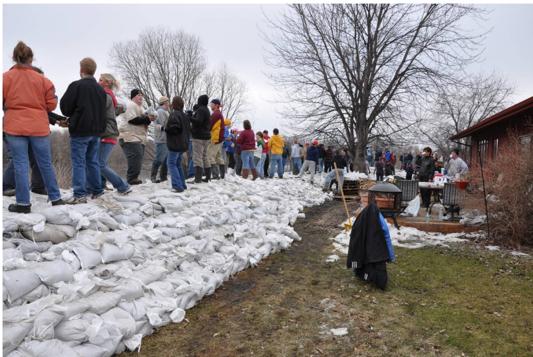
Picture 1 – Thousands of residents from the region assisted with building miles of sandbag levees in 2009.
